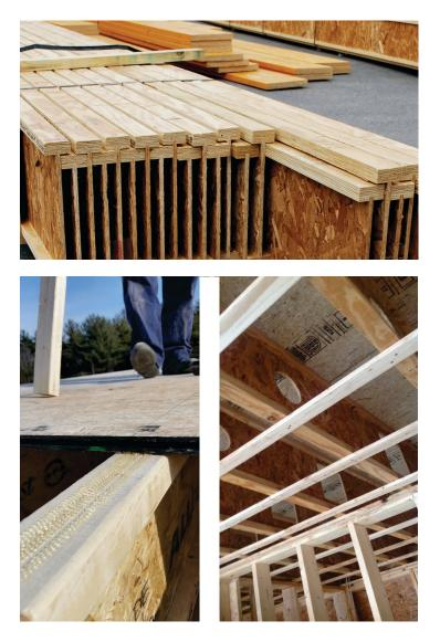
**Pre-applied sub-floor adhesive is the next costefficient step in improving the framing process.** National Lumber invested in the specialized equipment, training, and refinement of the process for pre-applying adhesive in our own manufacturing facility.
